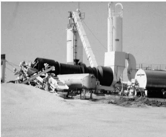
Dryer-drum Knockout Box
