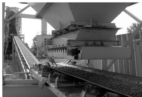
Cold elevator leading into the dryer
