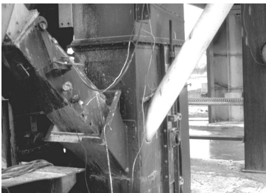
Base of the Hot Elevator
