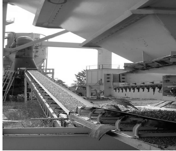
Batch Plant Cold Elevator
