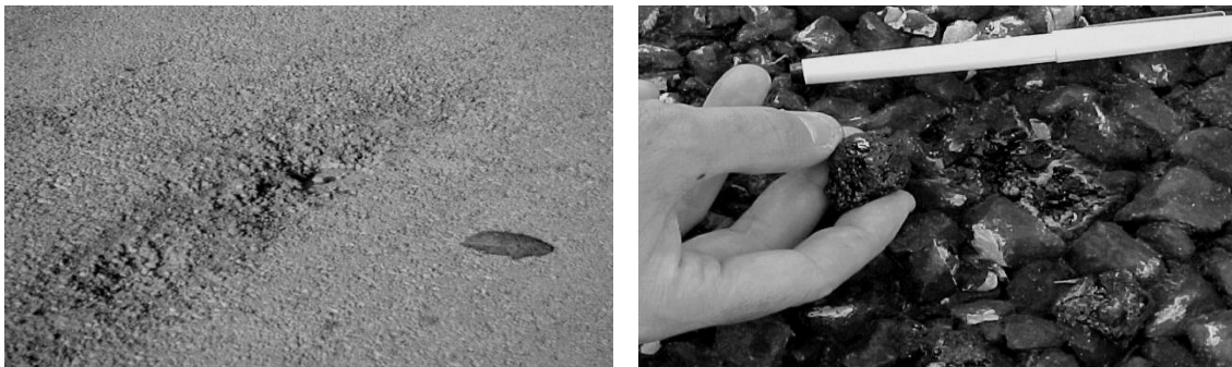
Effects of Liquid Asphalt Binder Stripping
