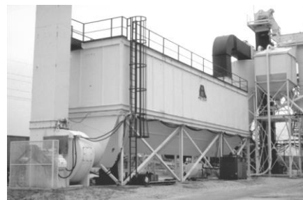
Secondary Baghouse Dust Collectors
